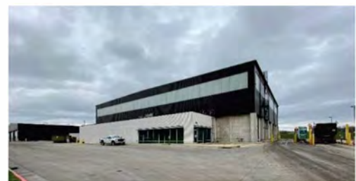
Figure 1: Morse Road Transfer Station
