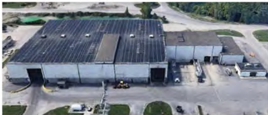
Figure 2: Jackson Pike Transfer Station
