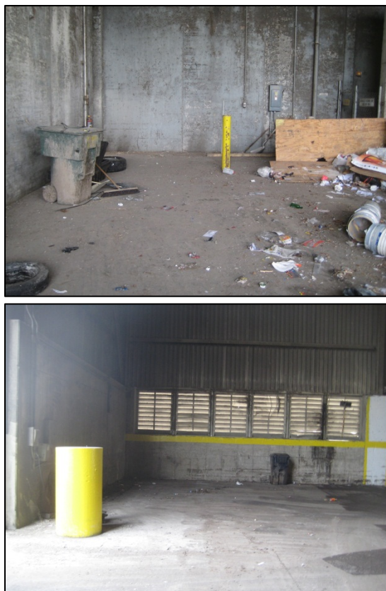
Figure 1 – Sorting Locations at Transfer Stations
