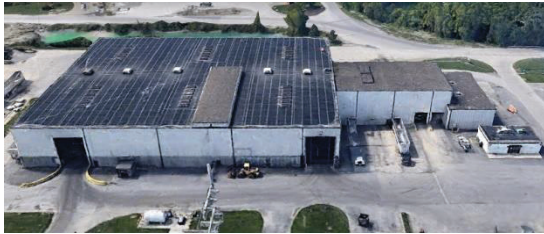
Figure 2: Jackson Pike Transfer Station
