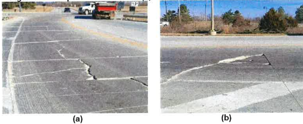
Figure 2. Example of Divided Slab (a) and Diagonal Crack with Punchout (b)
