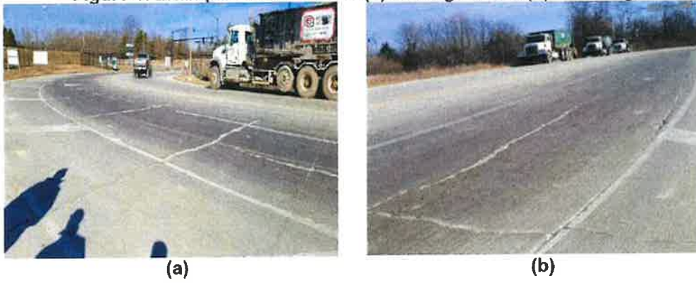
Figure 2. Example of Divided Slab (a) and Diagonal Crack with Punchout (b)
